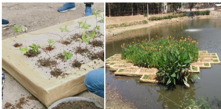
Figure 1: construction of floating treatment
